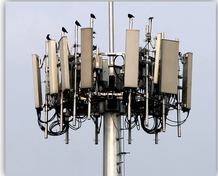
3 sectors, 4 vertical arrays per sector
